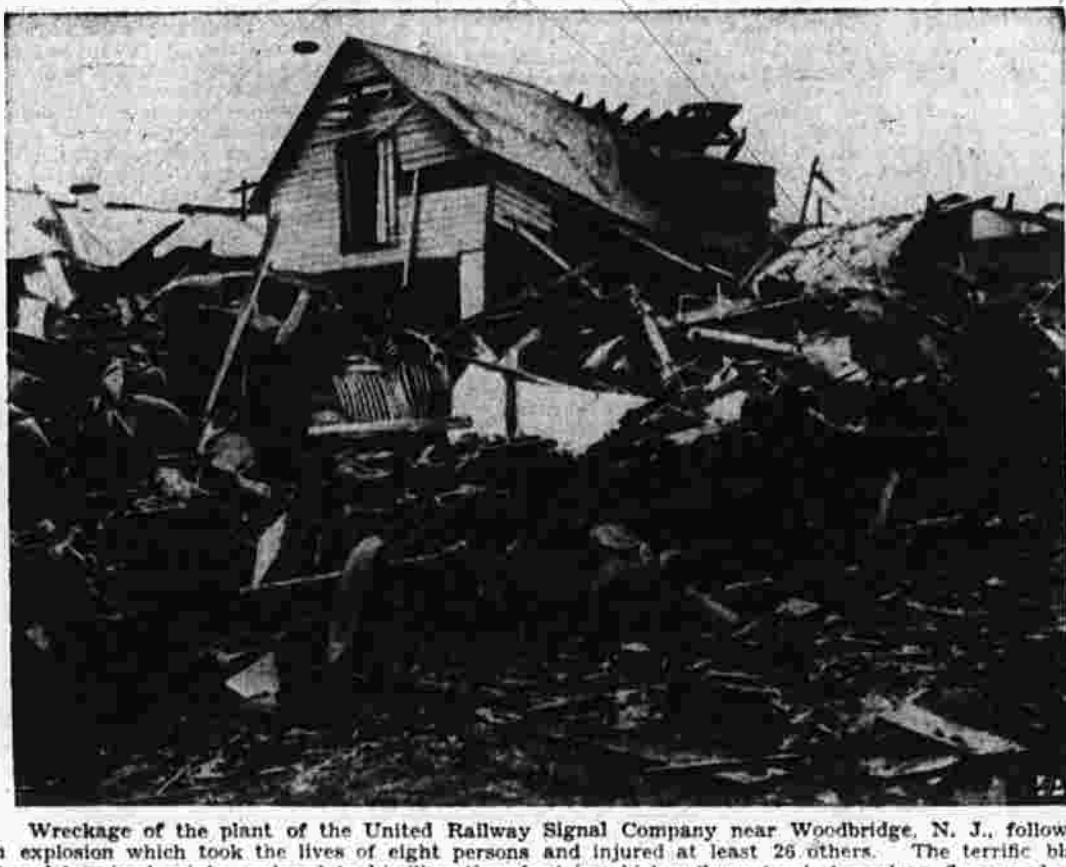
Wreckage of the plant of the United Railway Signal Company near Woodbridge, N. J., following an explosion which took the lives of eight persons and injured at least 25 others.
